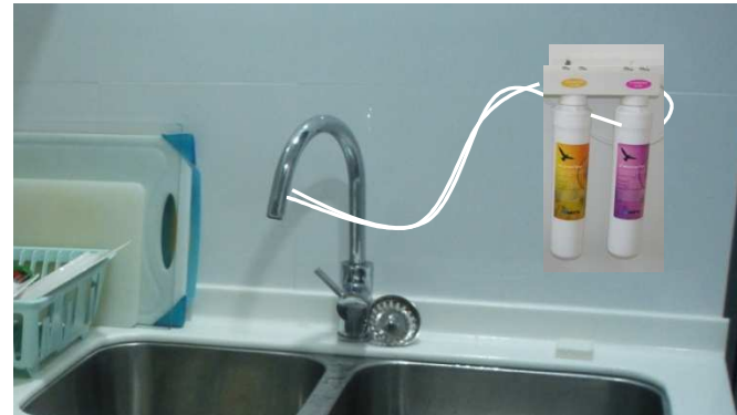
Kwik-Change™ unit fixed to the tile using double-sided tape
