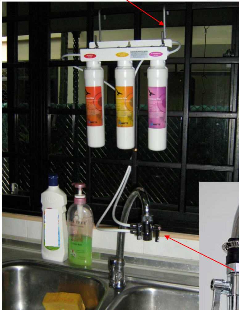
Kwik-Change™ unit is hung to window grille using hooks
