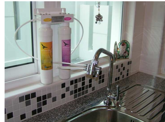
Filtered water flows through this outlet when lever is turned clockwise
